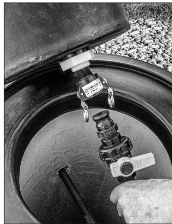
Float valve tub disconnected.
