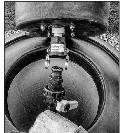
Floatless valve tub disconnected.
